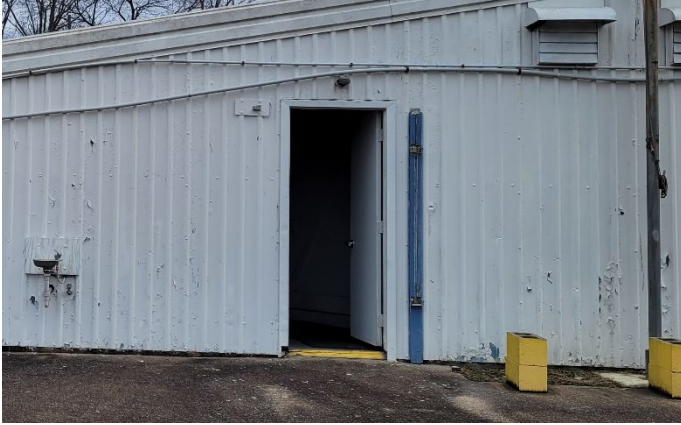
Metal Cladding on the West Elevation
