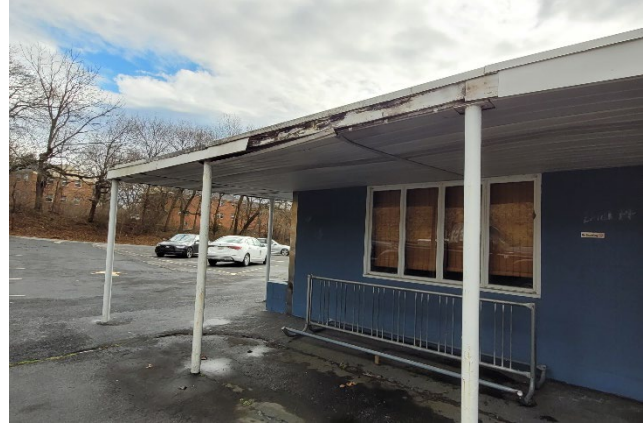
Deteriorating Fascia on the East Elevation
